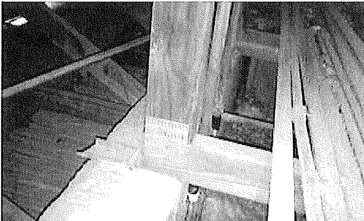
Roof to Wall Connection – Clips
